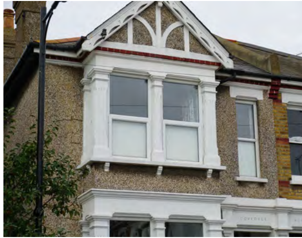
Inappropriate pebbledash render and uPVC windows
