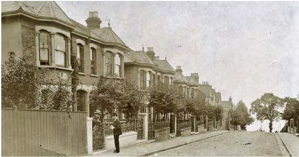
Victoria Road in the late-19th/early-20th century, looking south, showing semi-detached houses in brick, with double-height bay windows with timber sashes, and boundary walls topped with railings
