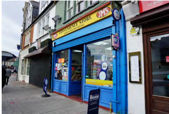
Unsightly roller shutter and garish colours and signage to a shop front
