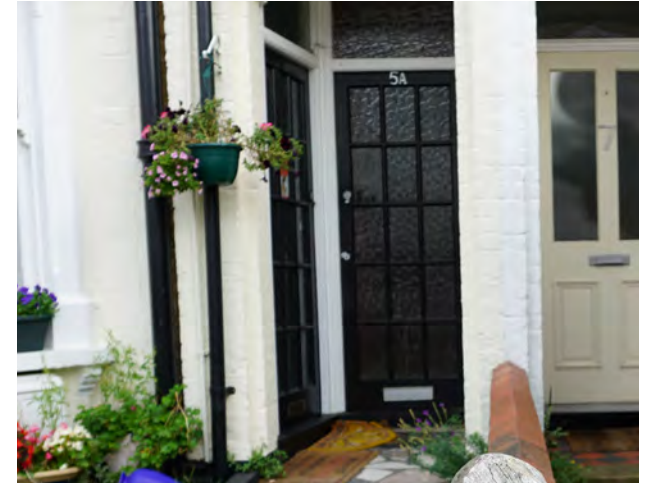
Additional door inserted within a recessed porch for the conversion of a house to flats
