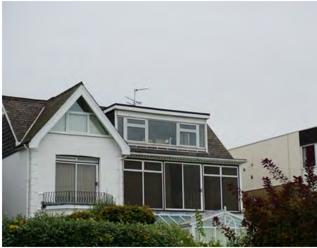
Inserted large dormer and picture windows
