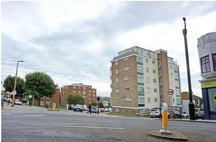
Large scale blocks of flats to the east of the Conservation Area on Grand Drive
