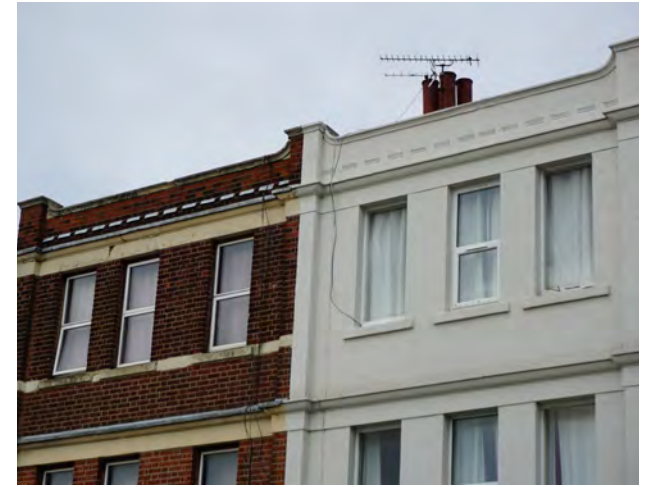
uPVC windows on upper floors of shops
