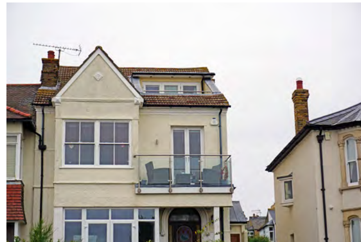
Glazed balustrade to balcony
