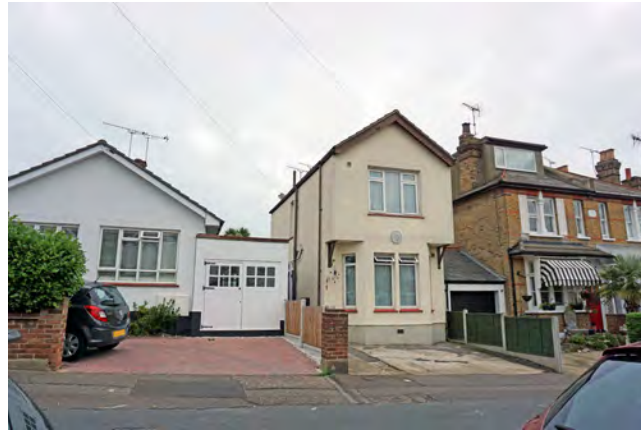
Driveways converted from front gardens, with poor surfacing and lacking planting
