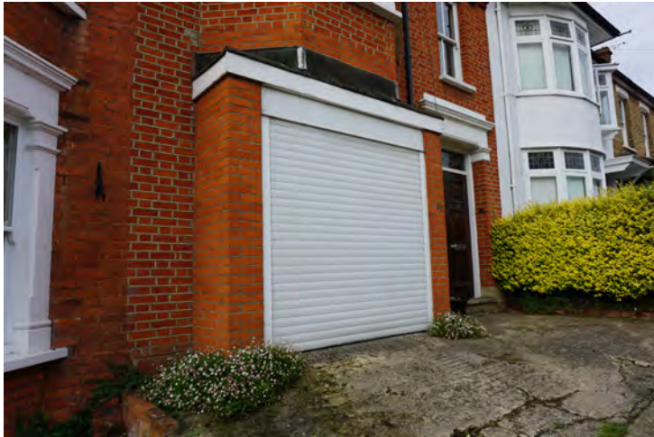
Ground floor garage inserted pre-1983 in the position of an original bay window
