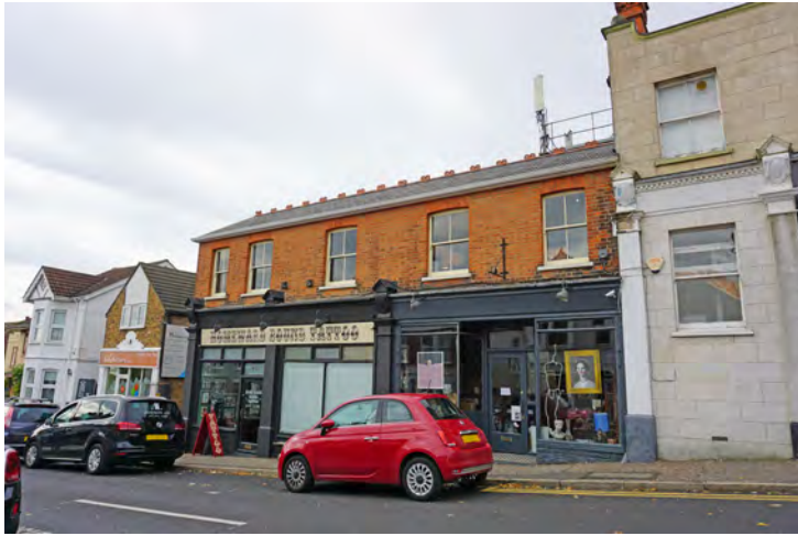
Good shop fronts and well-preserved range to the rear of Stuart House
